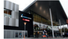
Åkersberga Centrum, Stockholm Citycon's GLA 28,200 sq.m. Anchor tenants ICA, Systembolaget
